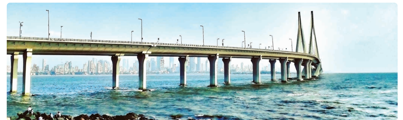
Bandra Worli Sea Link, Mumbai (Tata Steel's state-of-the-art durable LRPC strands and Tisco reinforcement bars were used in the construction)
